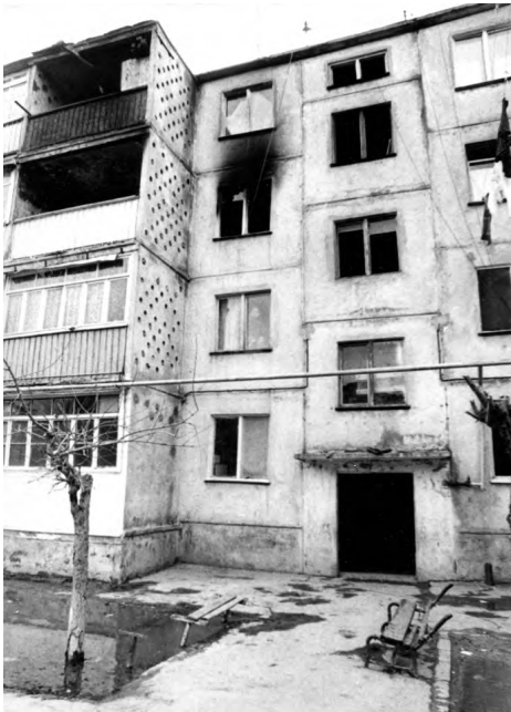
A destroyed and burnt building where Armenian families lived before the massacre in Sumgait (February 27-29, 1988).
